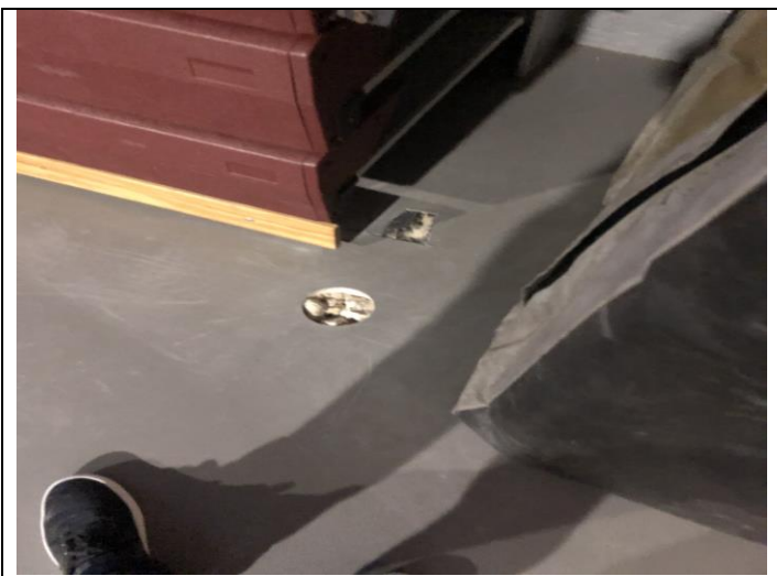
3. View of concrete sample location.
